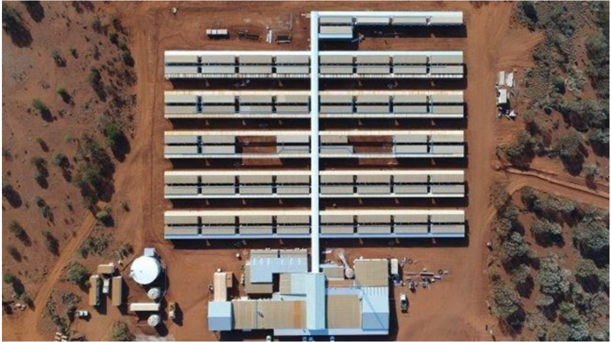
Figure 2: Installation of the accommodation village
