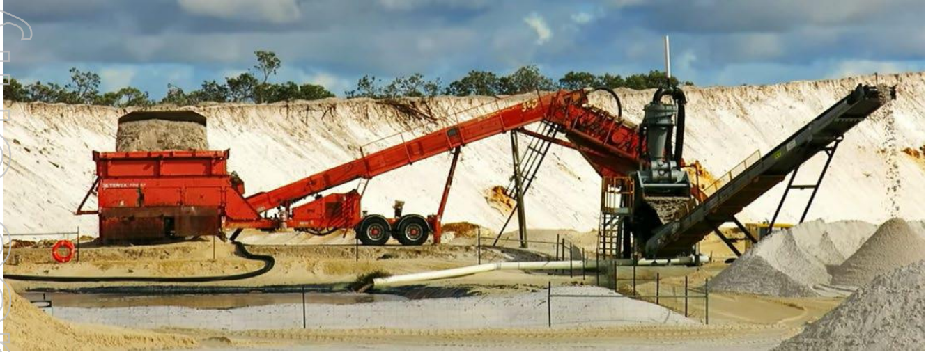
Urban's Maralla Rd Silica Sand Mine with silica sand washing plant in operation.
