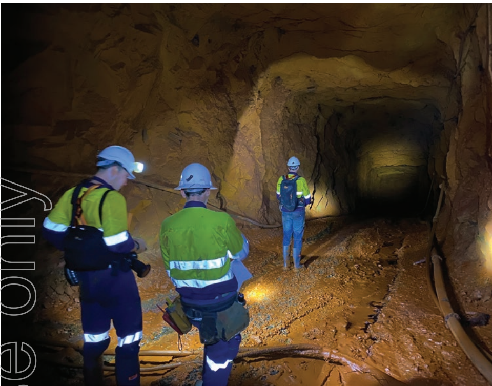
Bellevue technical staff inspecting the recently exposed main decline at the Bellevue underground mine during dewatering activities.
