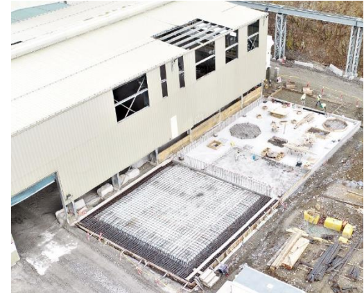
New Tailing Filter Civils
