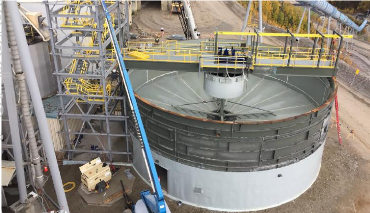
New Tailing Thickener construction
