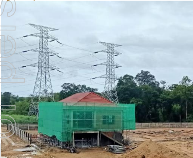
Figure Six | Substation Civil Works
