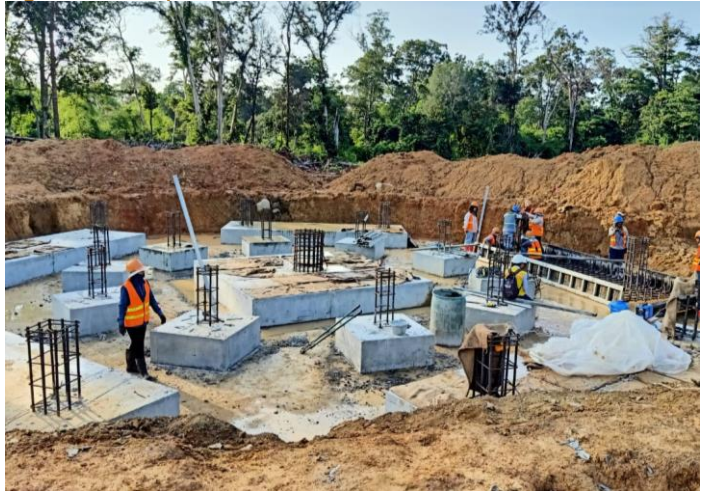
Figure Thirteen | Float Cell Foundation
