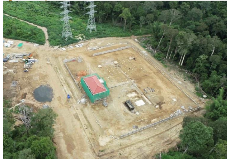
Figure Seven | Substation Civil Works Aerial view
