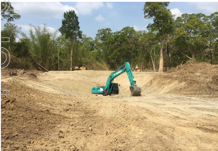
Figure Sixteen | Process Plant Sediment Pond
