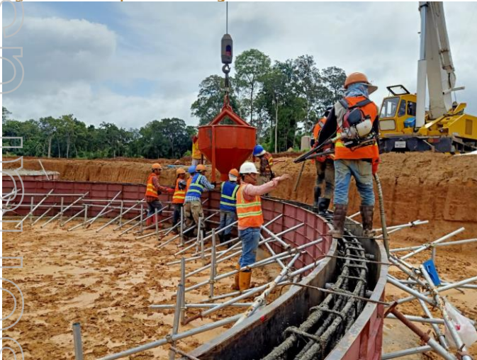
Figure Fourteen | CIL Tank Ring beams
