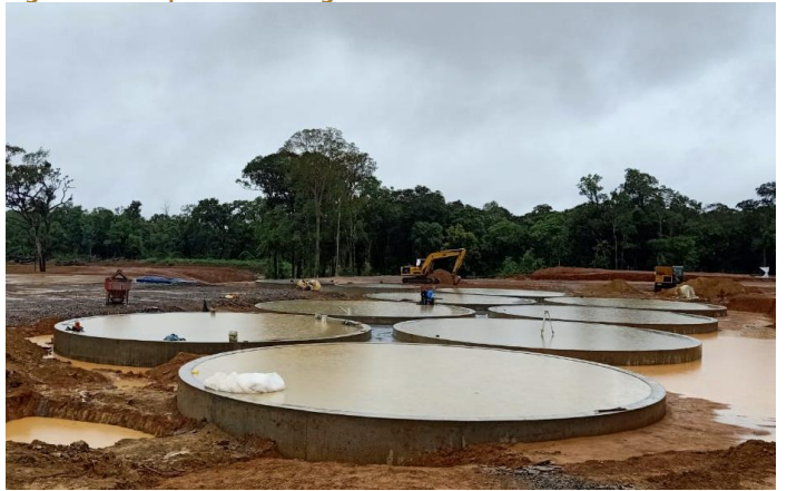
Figure Fifteen | CIL Tank Ring beams
