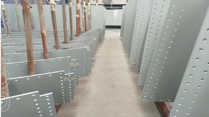
Figure Twenty Four | CIL tanks
