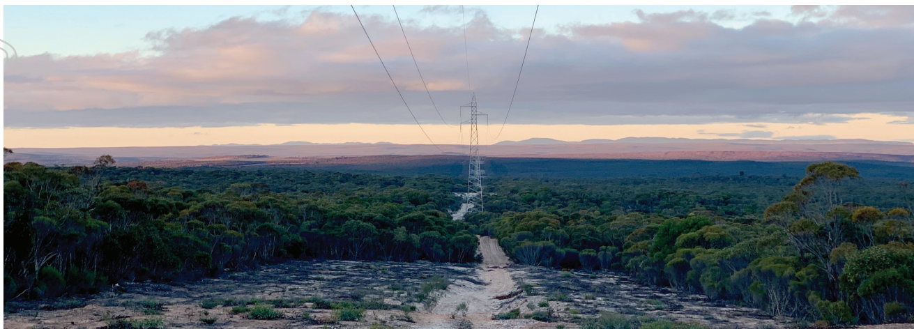
The Eyre Peninsula Link comprises a new 270 kilometre, high-voltage transmission line to be constructed from Cultana to Port Lincoln, via Yadrarie (Image- Jon Mussared)
