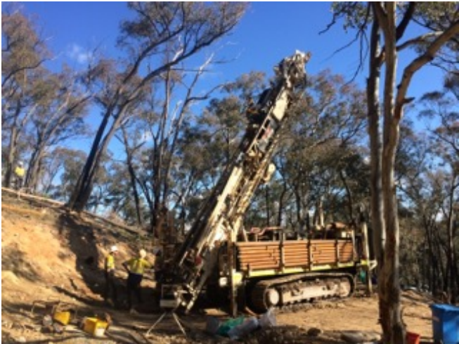
Figure 3: Drill rig in operation at the Main Ridge prospect, Basin Creek Project.
