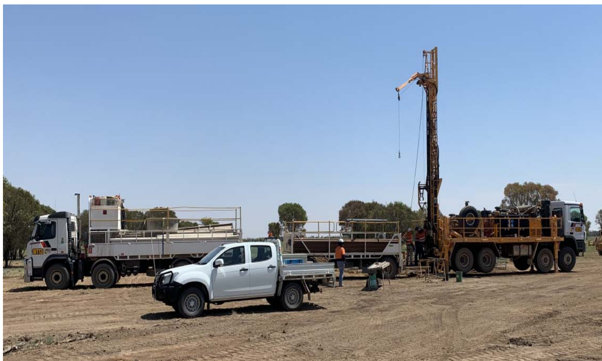
Figure 2: Drill rig at site BCP2
