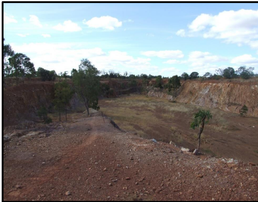
Figure 4: Lucky Break Gold Mine partly backfilled with tailings (looking north). Pit excavated to original depth of 15-30m
