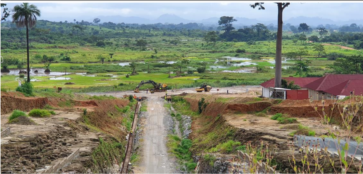
Figure 8: Storm water drainage construction
