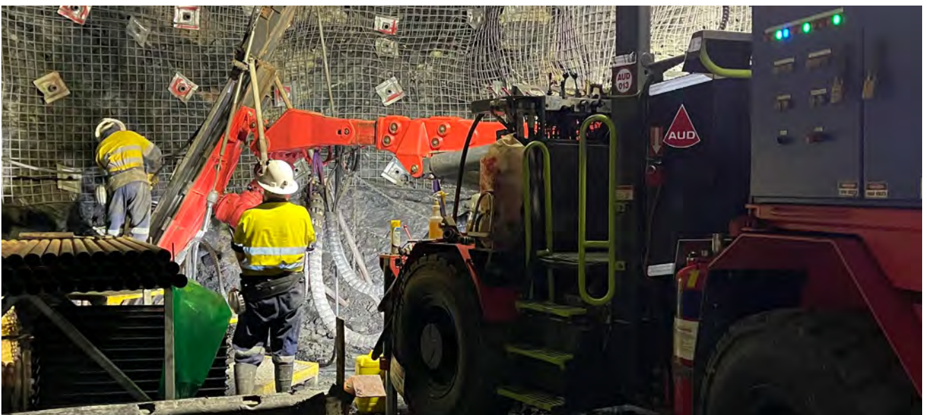
Figure 3: Underground Diamond Drilling from the 1445 SP
