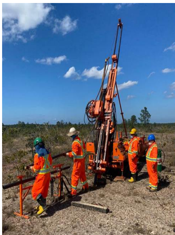
Diamond Drill Rig
