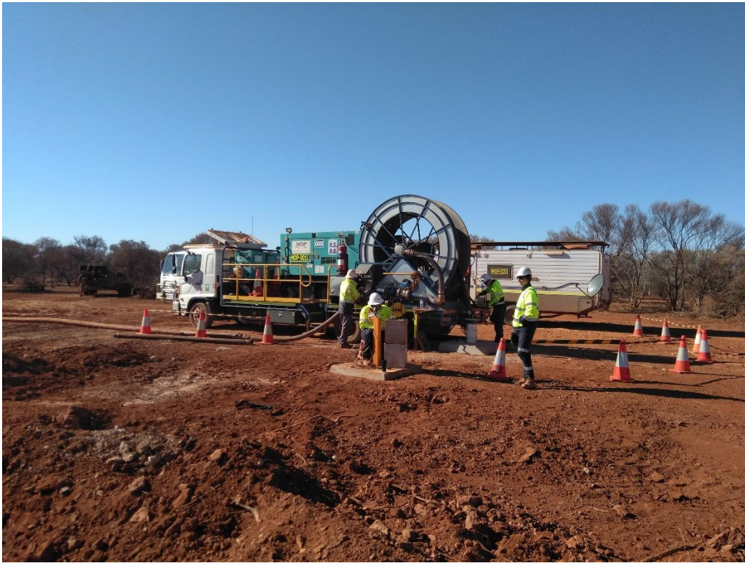
Figure 6: Water Production Bore Pump Testing
