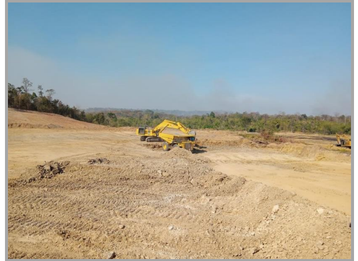
Figure 22 | Progress of Excavation works
