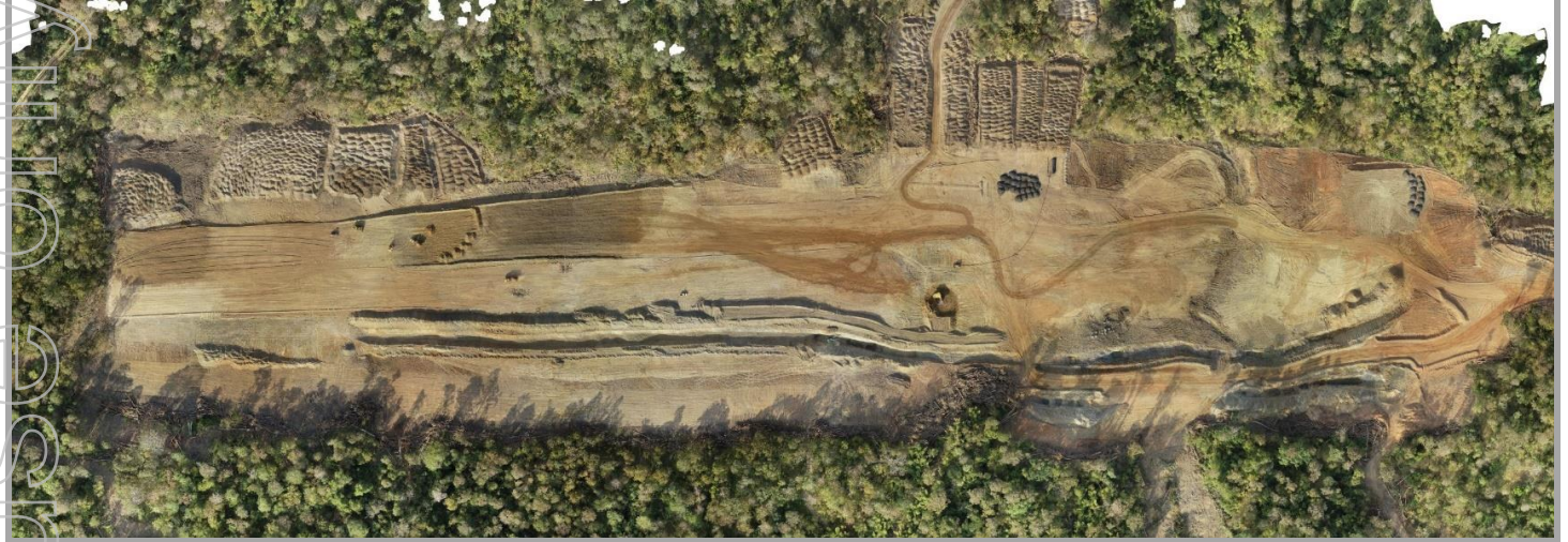
Figure 20 | Tailings Dam Footprint Cleared, Topsoil stockpiled and Keyway cut
