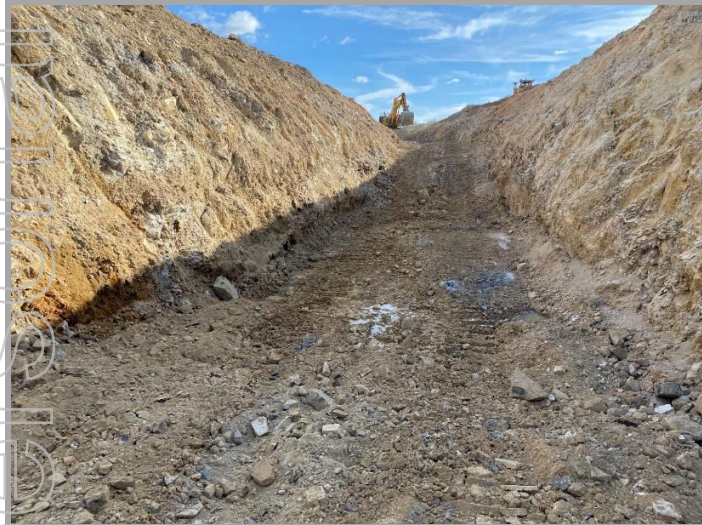
Figure 21 | Tailings Dam - Keyway Excavation works
