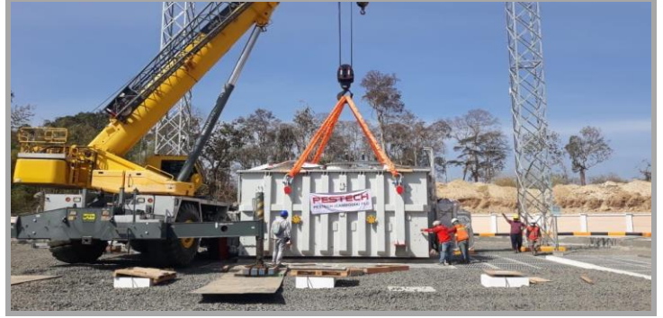
Figure 27 | Installation of Transformer
