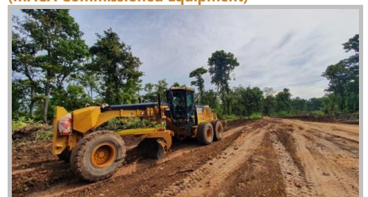
Figure 25 | Contractor Yard Clearing (MACA Commissioned Equipment)
