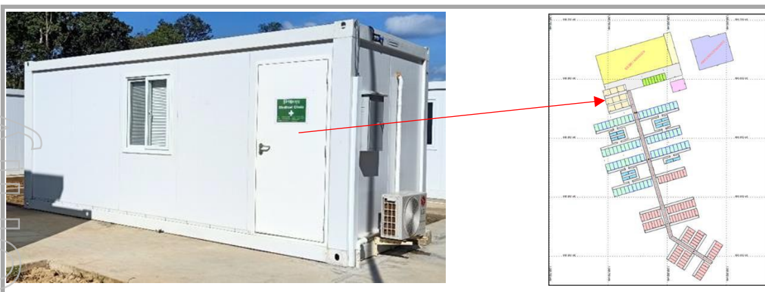
Figure 46 | Okvau Village Medical Centre now operational
