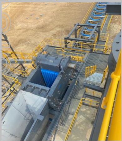
Figure 16 | Primary Crusher Installed
