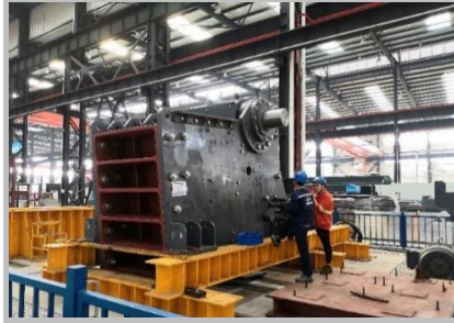
Figure 11 | Trial Assembly of Primary Jaw Crusher
