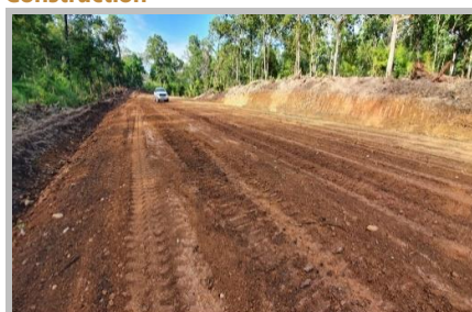
Figure 24 | Haul and Site Access Road Construction
