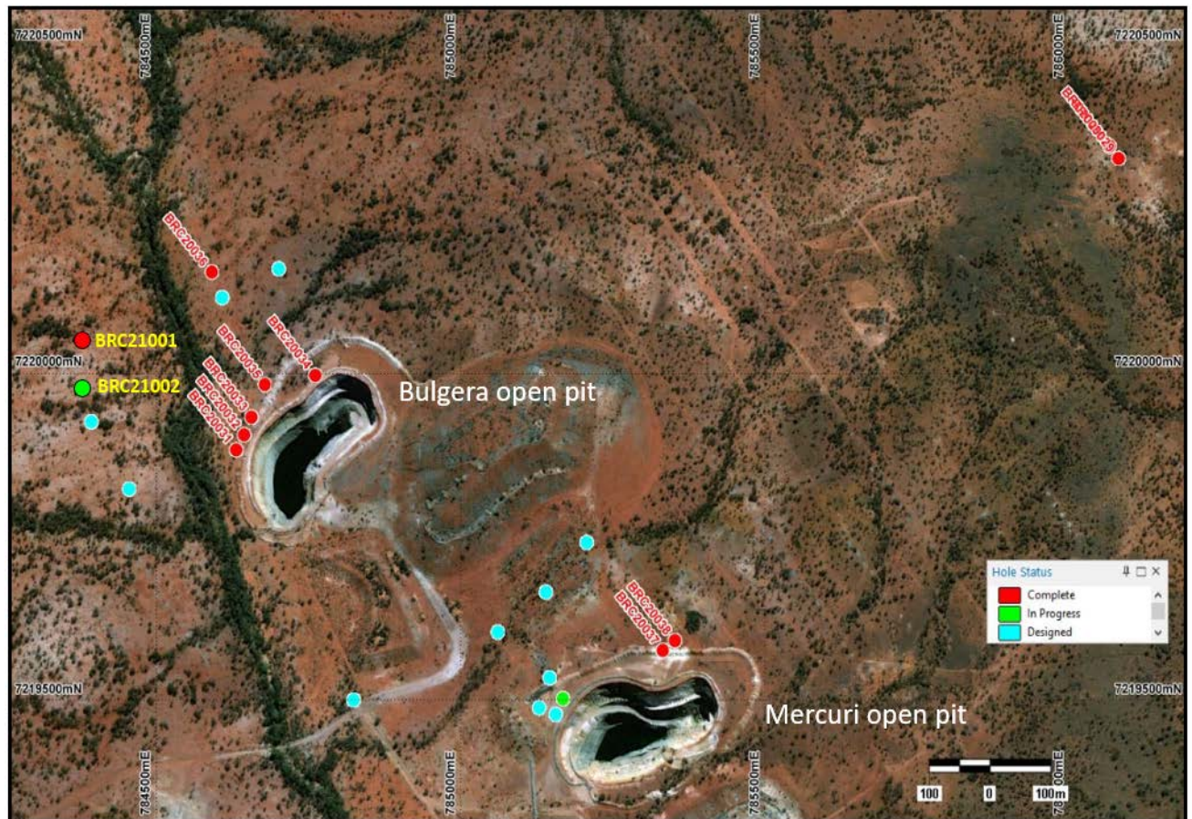
Figure 4 - Status of RC drilling at Bulgera & Mercuri open pit areas as at 19 January 2021
