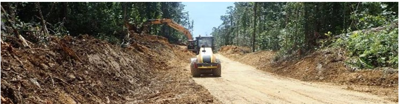
Figure 4: Construction of Road Infrastructure
