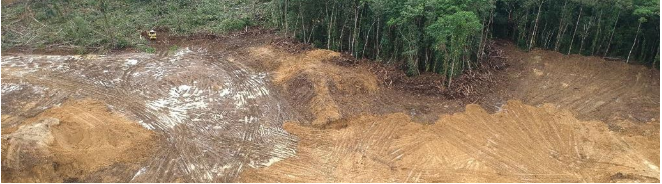
Figure 3: Plant site Land Clearing
