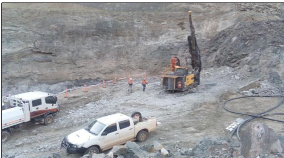
Plate 1 Granny Venn Pit Floor RC drilling at RL 380m.
