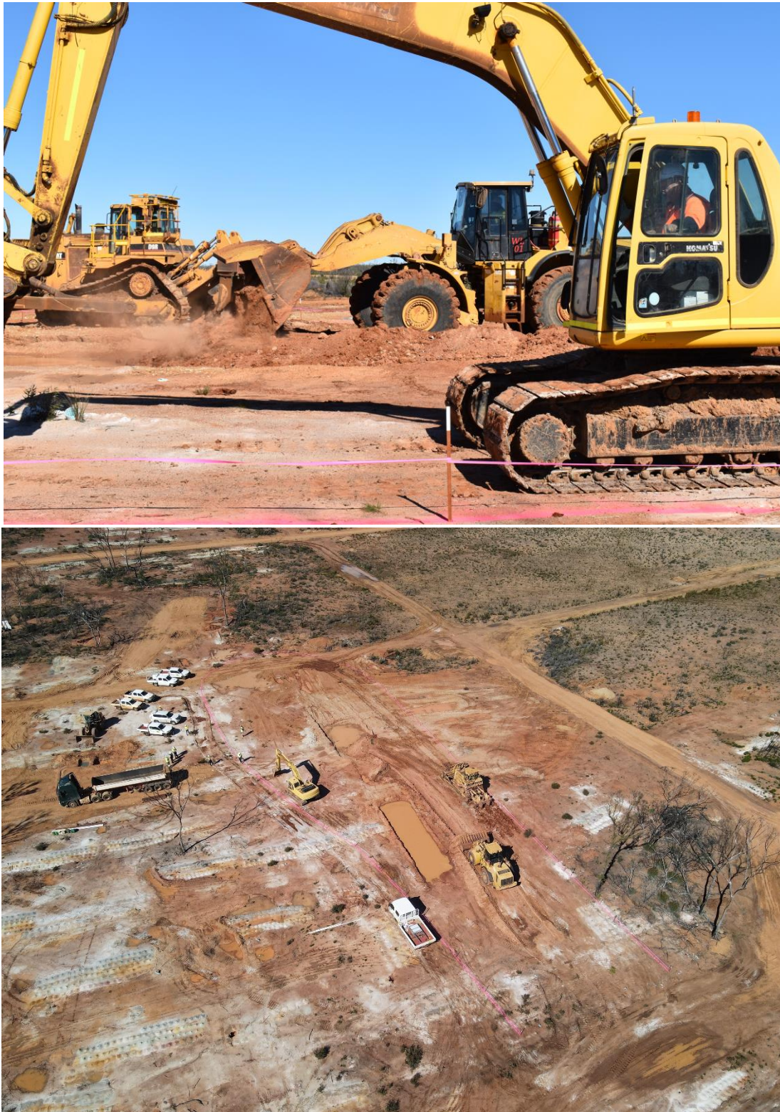
Figure 6: Earth-moving equipment -Top, Aerial view (From Above)
