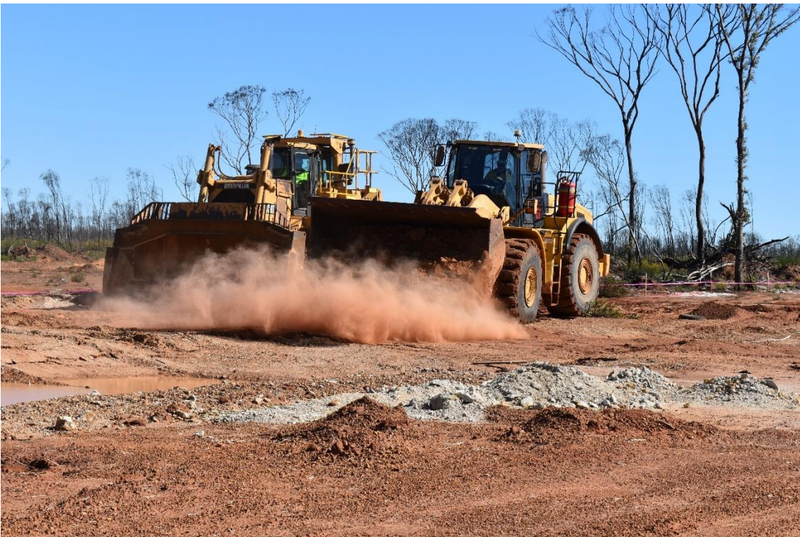
Figure 4: Dozer and Loader commence pushing back top soil at Bulk Sample Pit.
