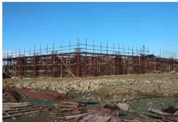
Column reinforcement for Electrostatic Precipitator
