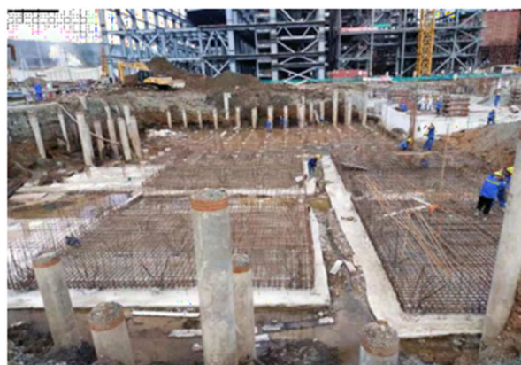
Foundations for ANI powerplant
