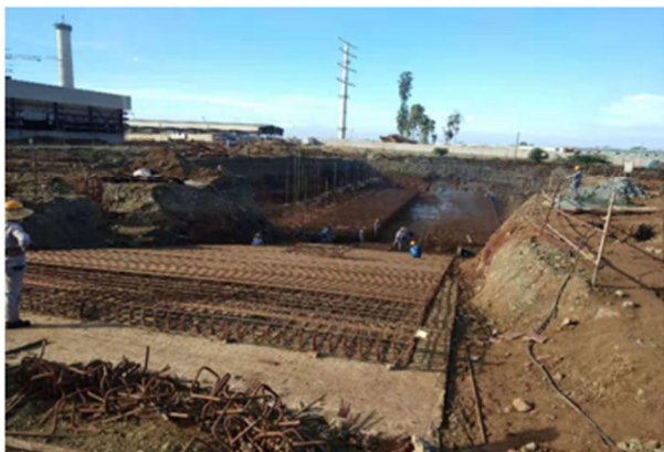
Foundations for Dry Ore shed
