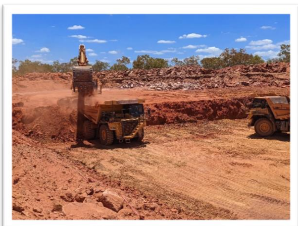
Figure 2: Waste mining by excavator and truck
