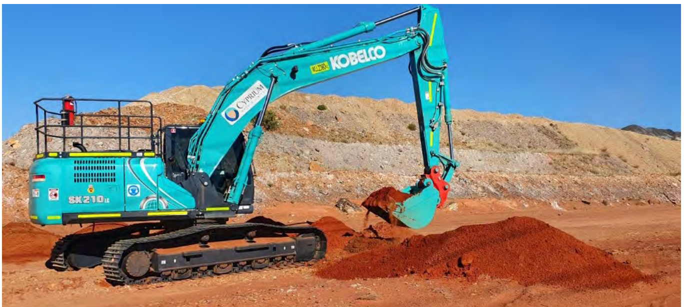
Image 6 | Commencement of the Nifty Geotechnical test pit with a 20t Excavator
