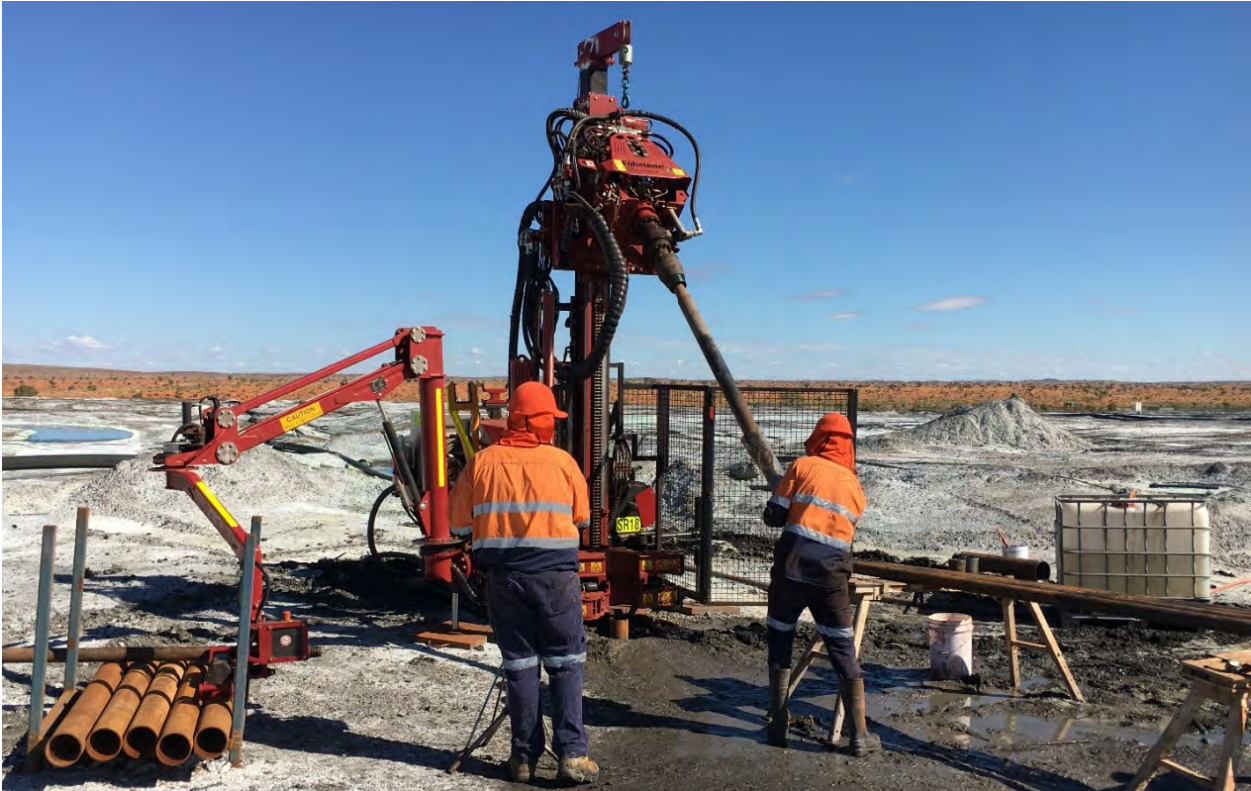
Image 1 | Sonic Rig at the Heap Leach Pads
