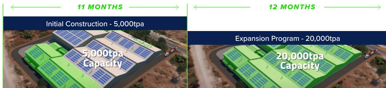
EcoGraf Kwinana-Rockingham Processing Facility
