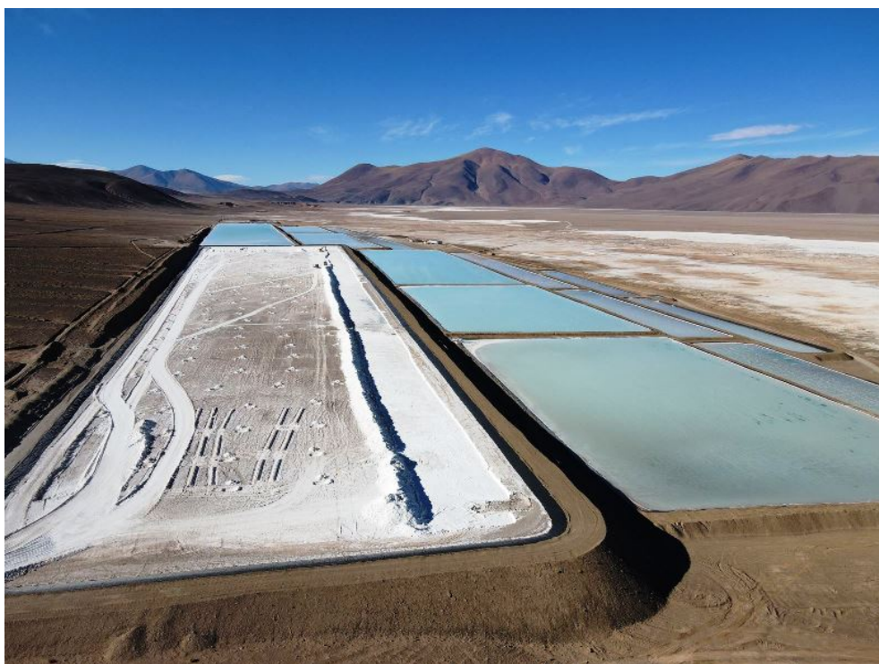
Figure 1. Rincon Lithium Project – Salt Harvesting Works
