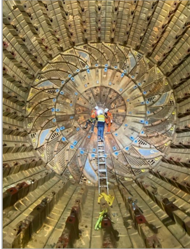
Figure 11 | Final mill liner segment installation
