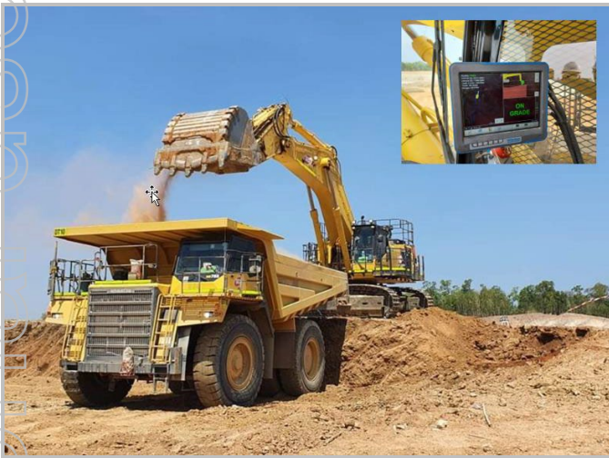
Figure 13 | The first ore load of Okvau. Block ID ST1_160_003G (Screenshot of APS shows the floor control on grade)
