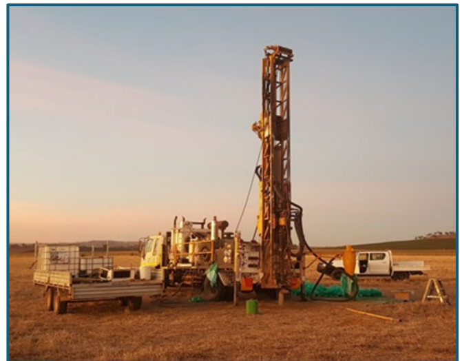
Figure 8: Drill rig in operation at Junee Project, NSW.
