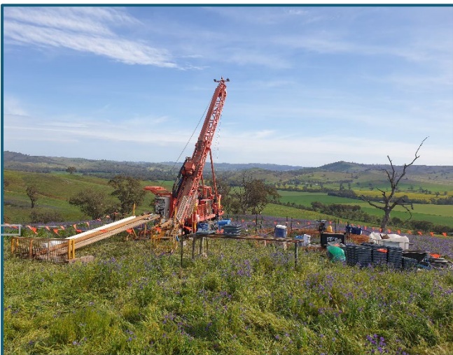
Figure 13: Diamond drill rig in operation at Junee Project, NSW.
