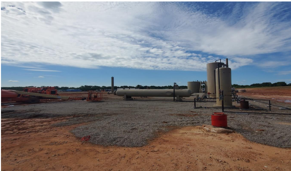
Figure 2. Jewell Well production facilities (tank battery and separators).
