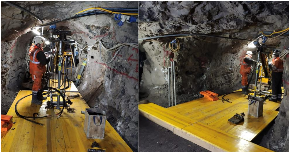
Figure 2: Diamec-230 Drill Rig Underground at Ponente
