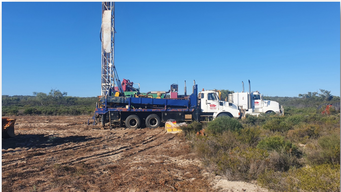
Figure 6 - Water Bore Rig onsite
