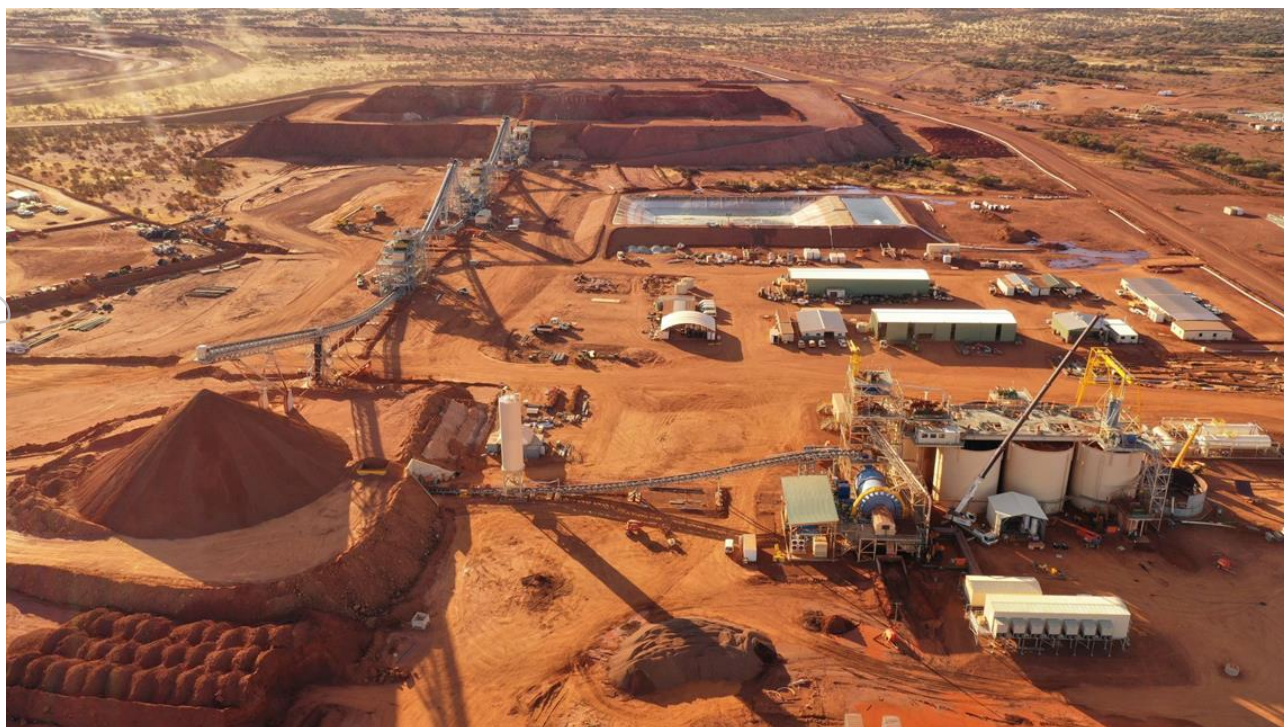
Figure 2: Karlawinda Processing Plant
