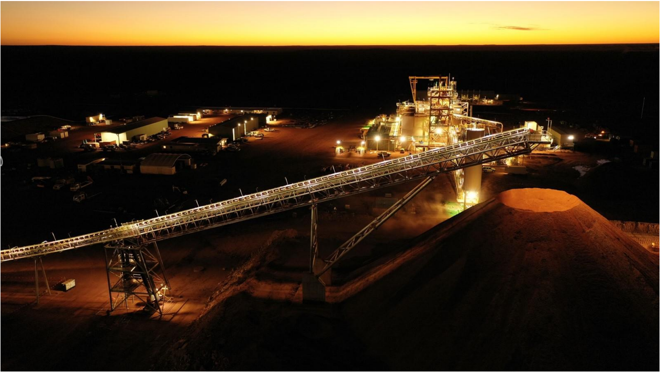
Figure 3: Karlawinda Processing Plant
