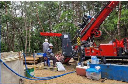
Drilling at Nettle, Deokon Project.
