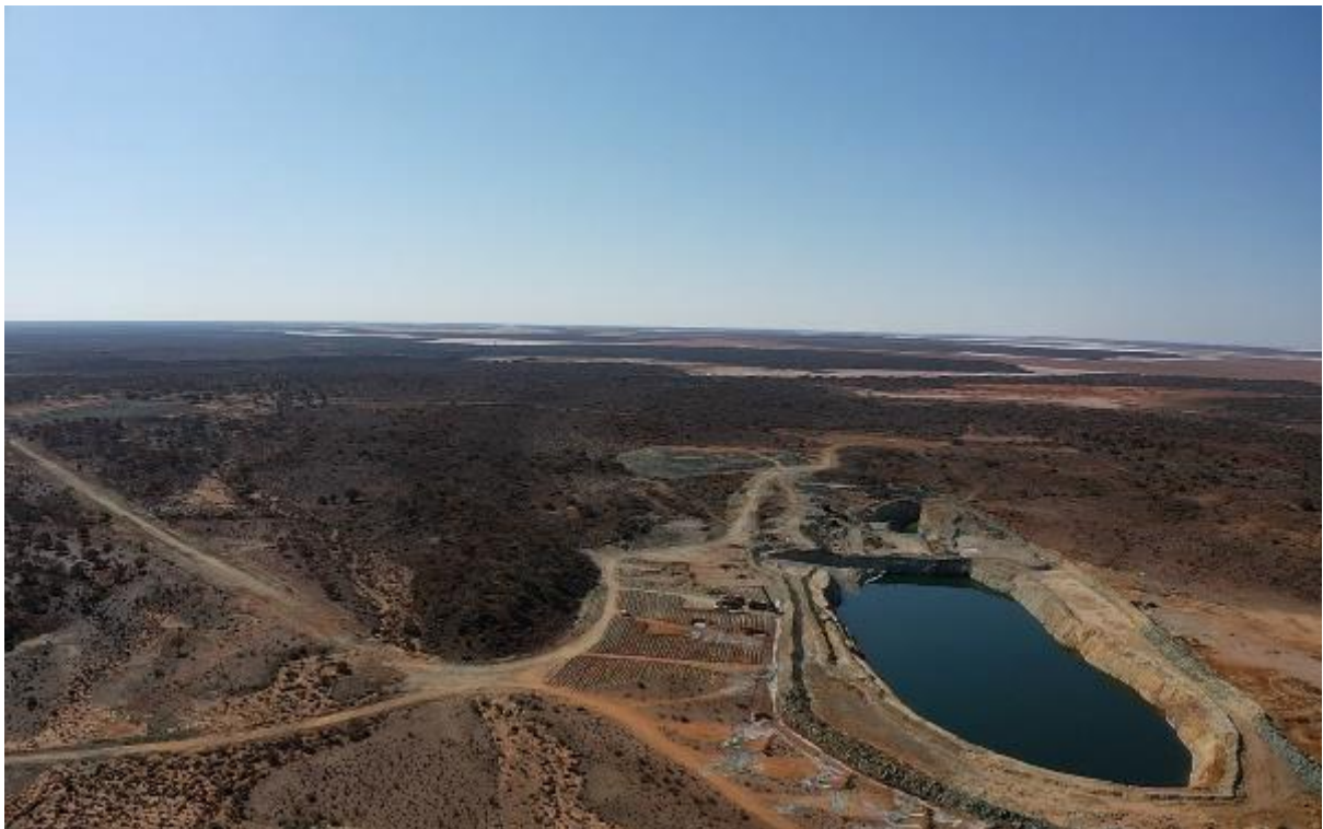
Devon Pit Looking north towards Red October
