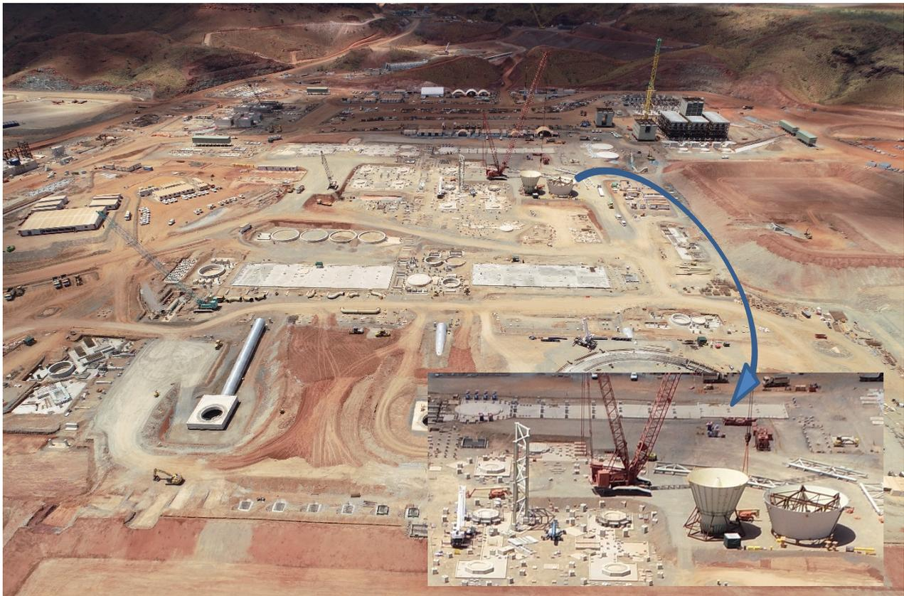
*First steel erected and cone sections assembled for the LFCU processing area.*
