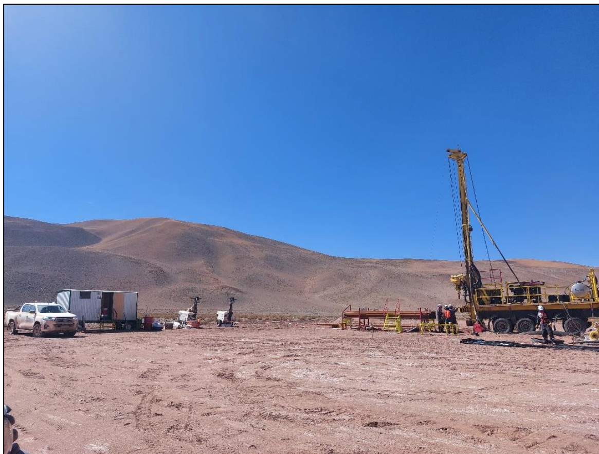
Bore well at Rana de Sal
