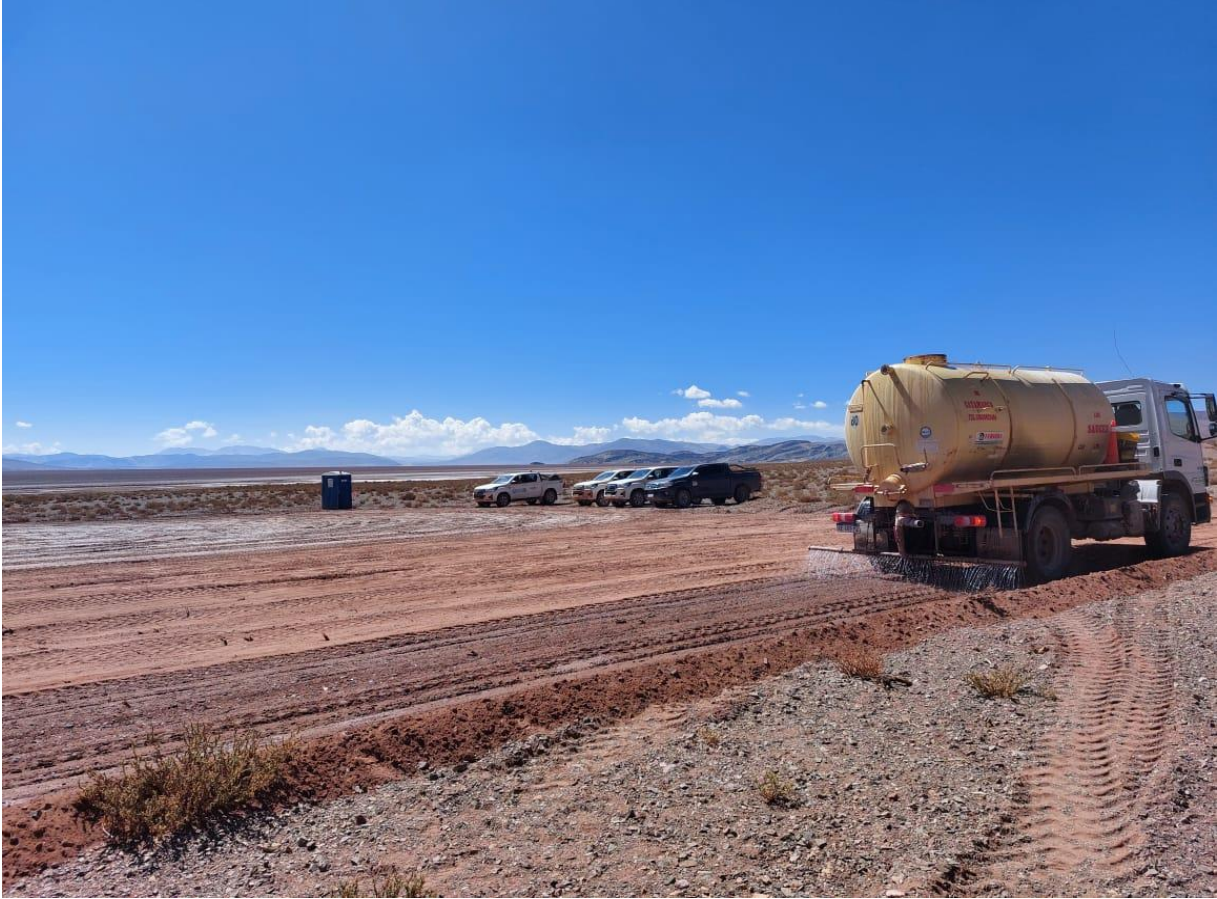
Construction of evaporation ponds at HMW Project
