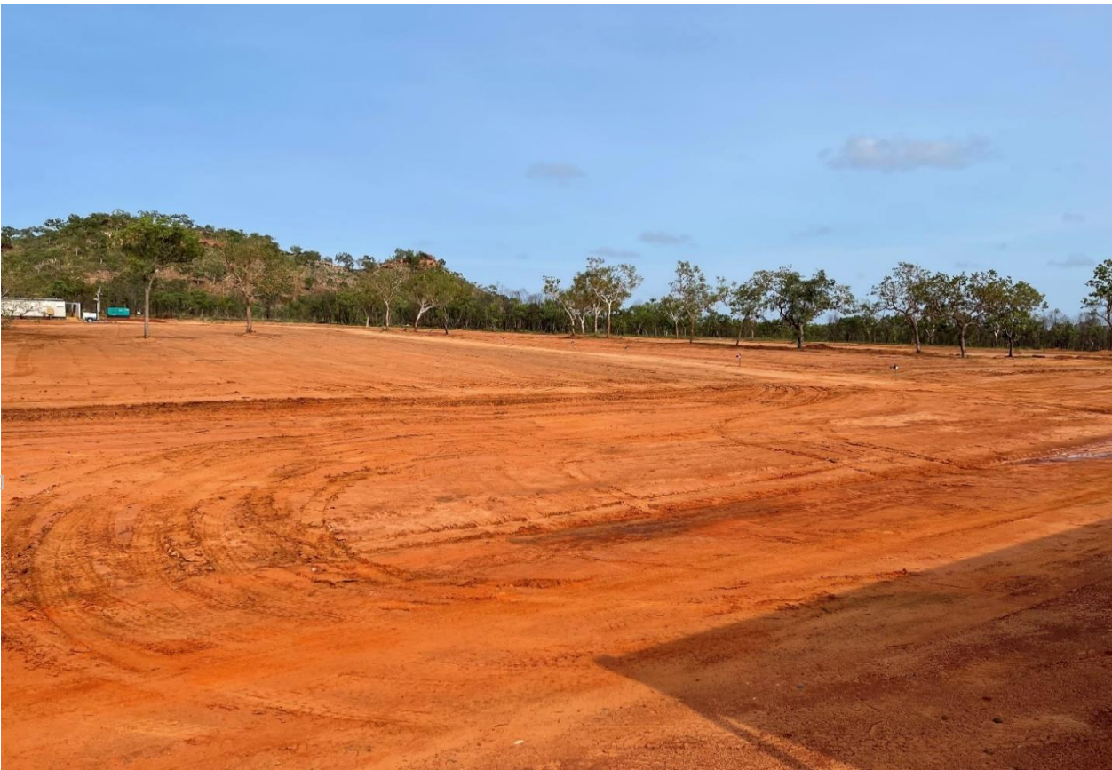
Figure 3: Thunderbird village accommodation site clearance activities
