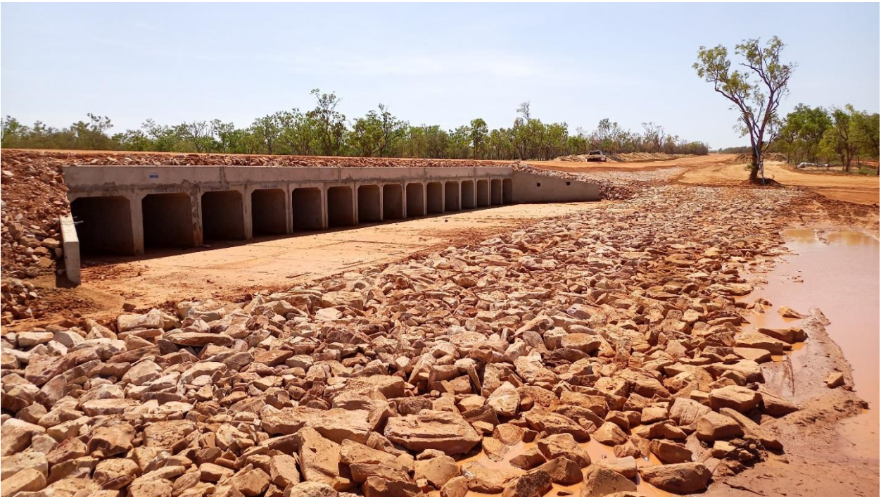
Figure 2: Thunderbird mine access road – culvert installation
