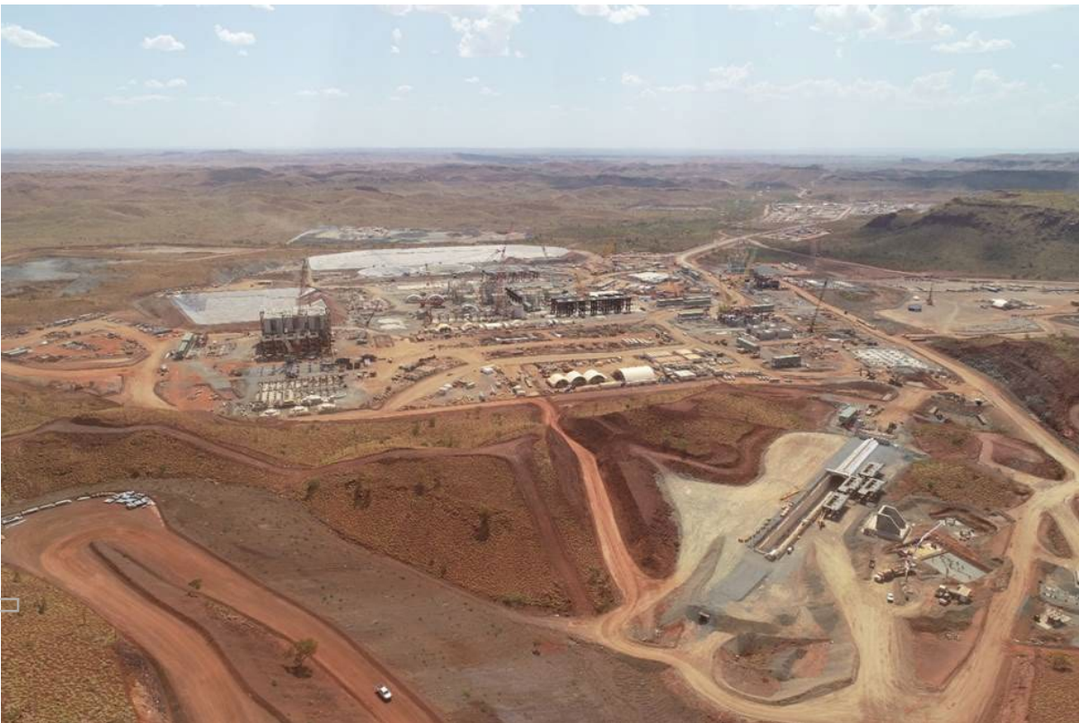
Image – Iron Bridge Wet processing facility progress update
