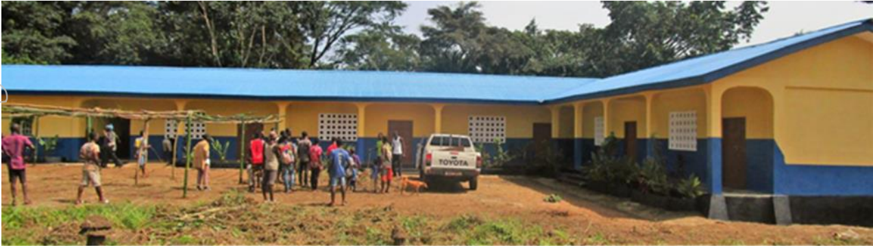
Completed Secondary School in Tongo Community
