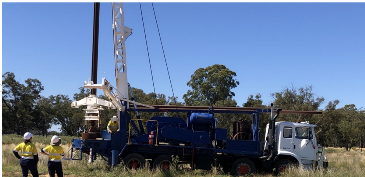
Figure 3: Platina Lead Drilling
