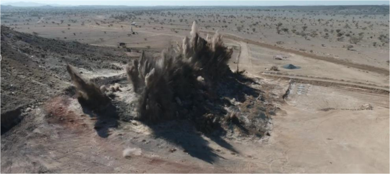
First controlled blast at Wash-hi Majaza site
