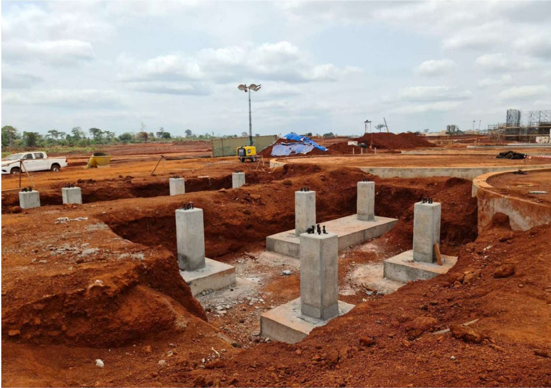
Figure 8: Abujar Gold Mine processing plant CIL ring beams and Pedestals poured
