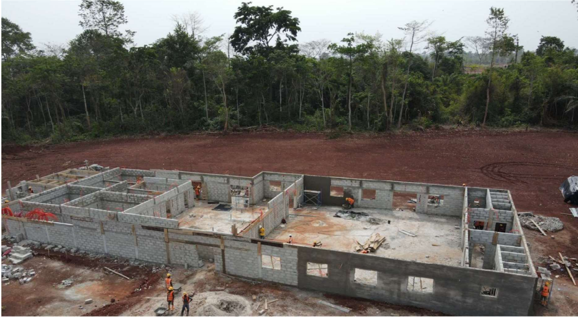
Figure 6: Abujar Mine Camp canteen building in construction
