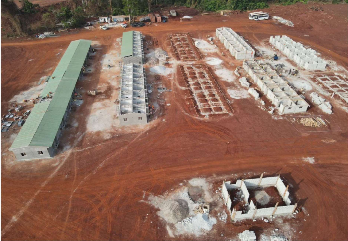
Figure 4: Abujar Mine Camp accommodation buildings in construction
