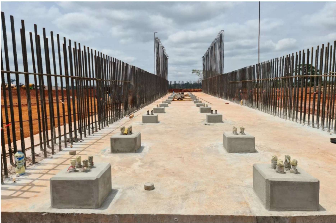
Figure 9: Abujar Gold Mine processing plant Reclaim – Conveyor CV02 Pedestals
