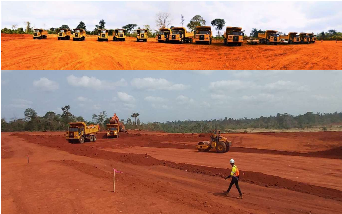
Figure 10: Tietto's dump truck fleet working at Abujar
