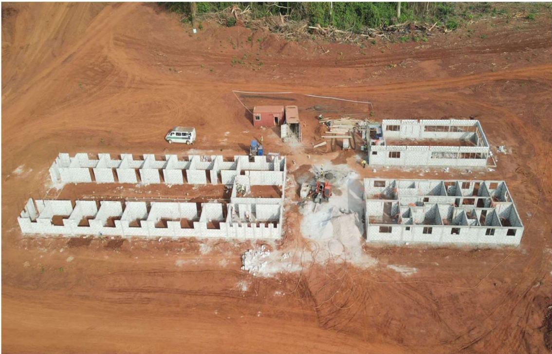
Figure 5: Abujar Mine Admin, Clinic and Training buildings in construction
