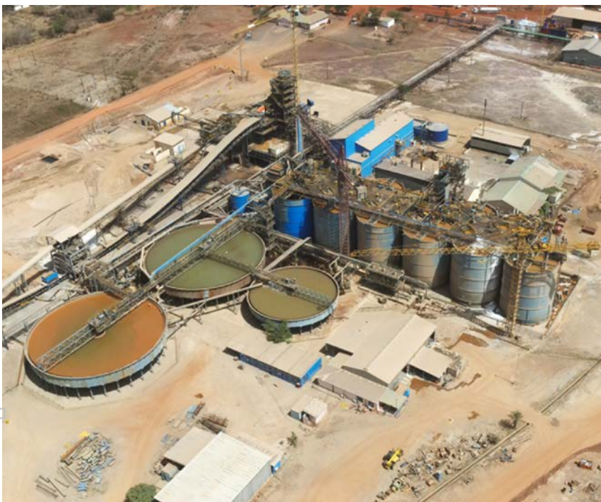
Pictured Left: Ball mill refurbishment and plant structural steel replacement Top: PhotonAssay lab technology to be installed at Morila (Pic Source: Chrysolab) Below: Morila Processing Plant
