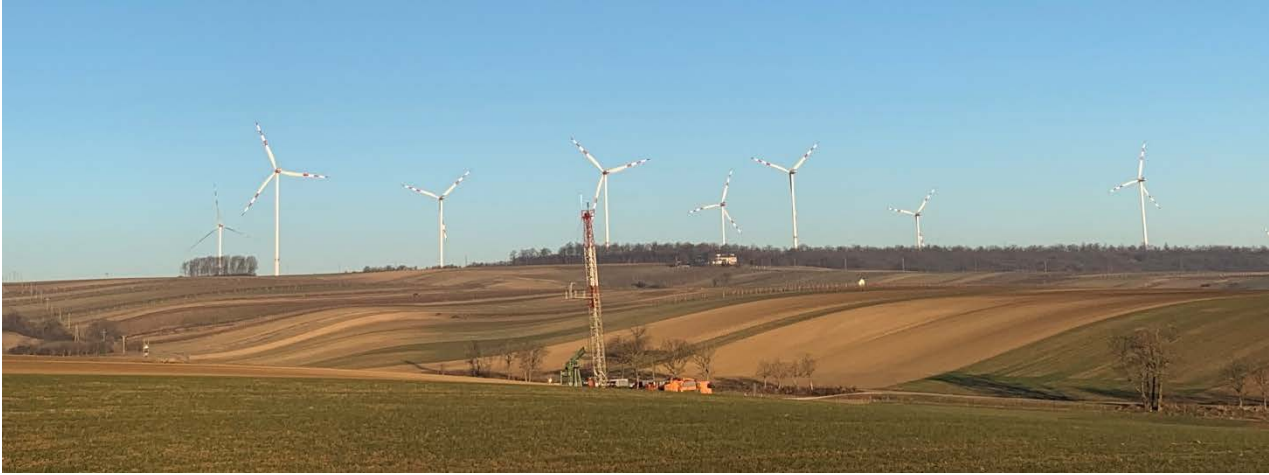
The RED workover rig W-102 which has been utilised for workovers in ADX' Vienna Basin Oil fields
