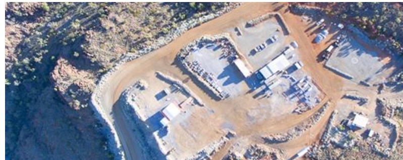
Northwest Queensland (Operating)
