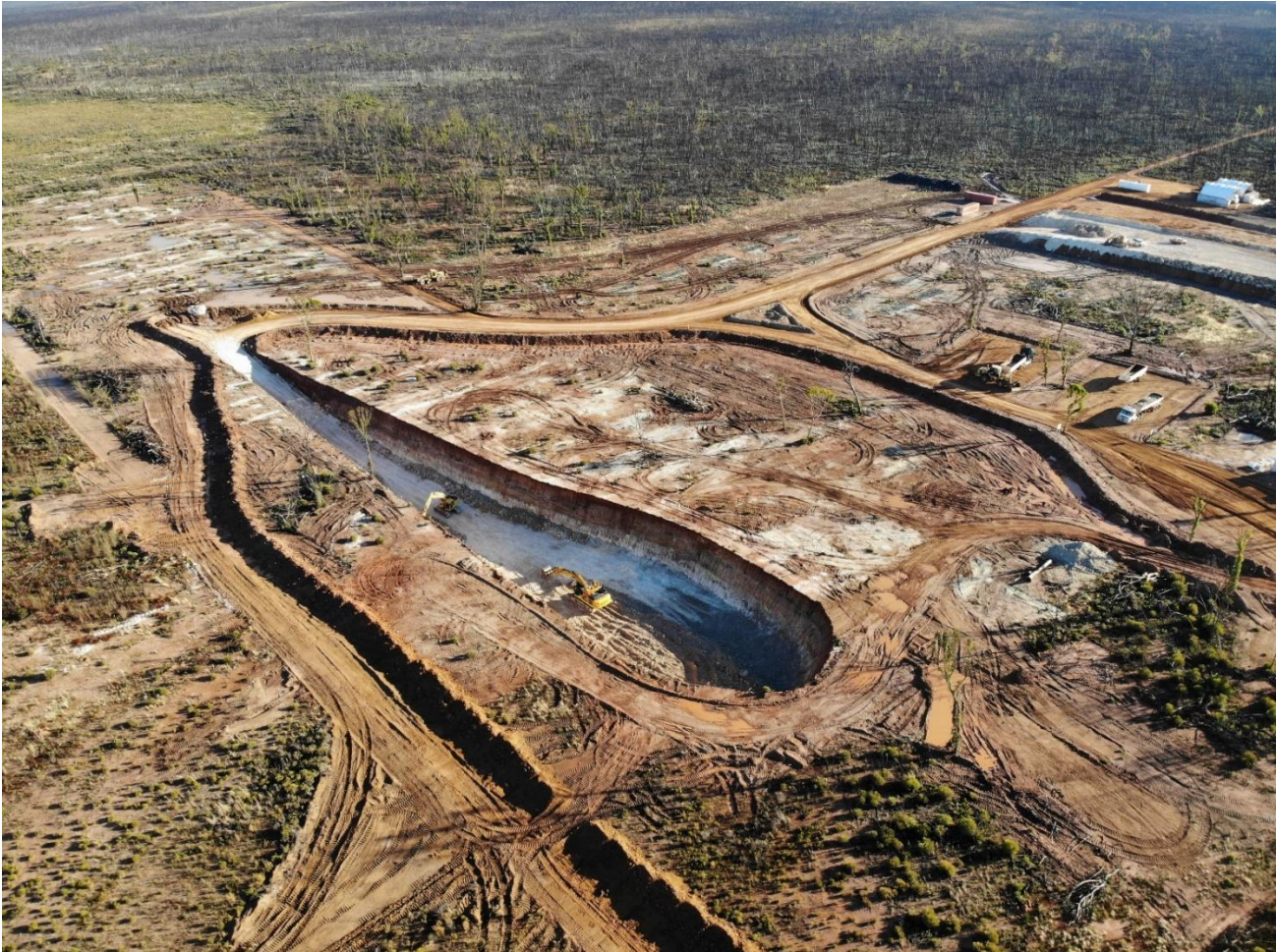
Figure 2: Aerial view of pit – Showing overburden almost removed prior to first ore exposure.
