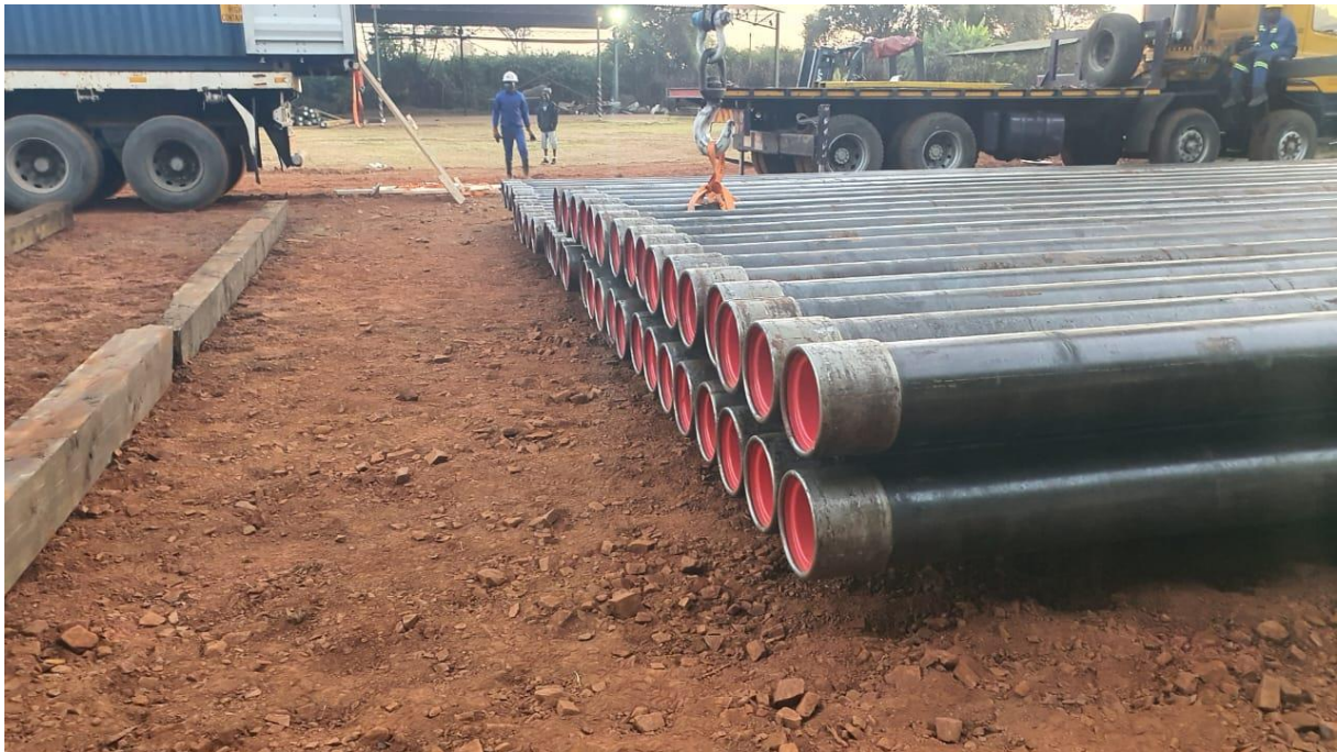
Figure 3 - Casing being prepared for racking and deployment to Mukuyu-1 wellsite
