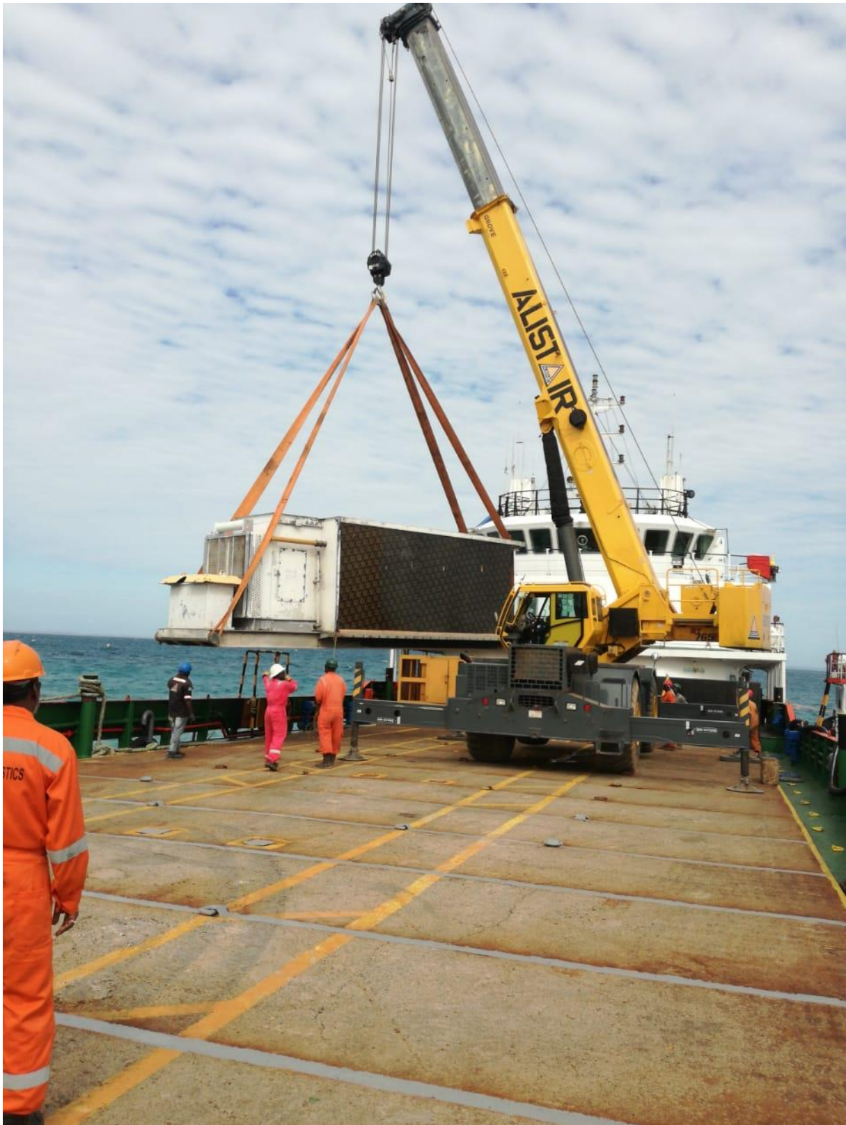
Figure 2 - First load out of equipment onto barge at Songo Songo Island
