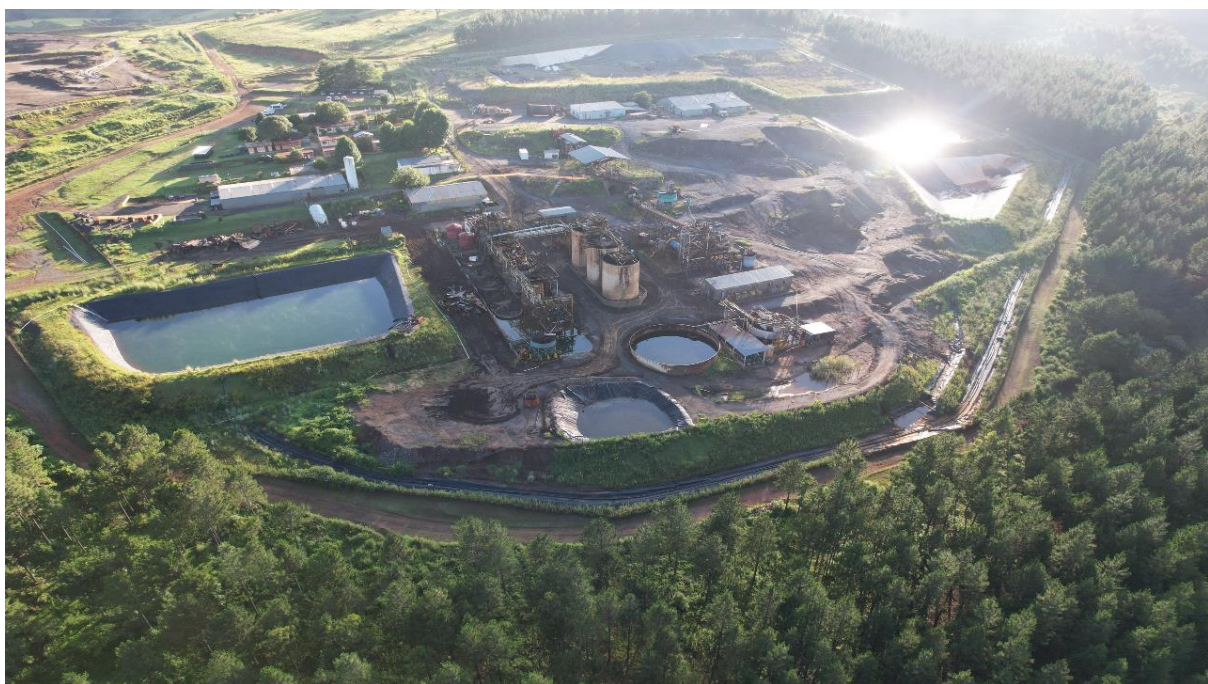
Figure 3: Existing Plant Drone View (post demolition of old sections)
