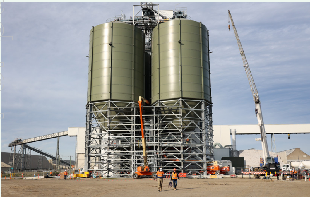
Geelong Cement grinding and storage facility, Vic
