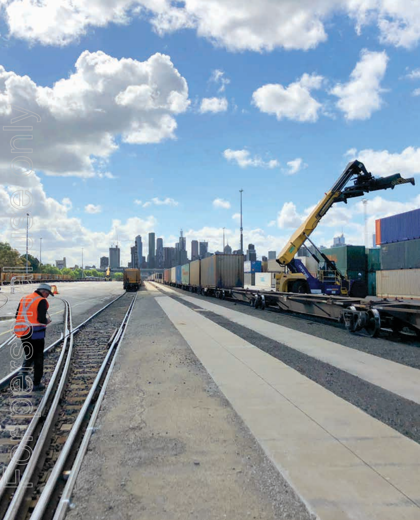
Track inspection, Melbourne, Victoria
