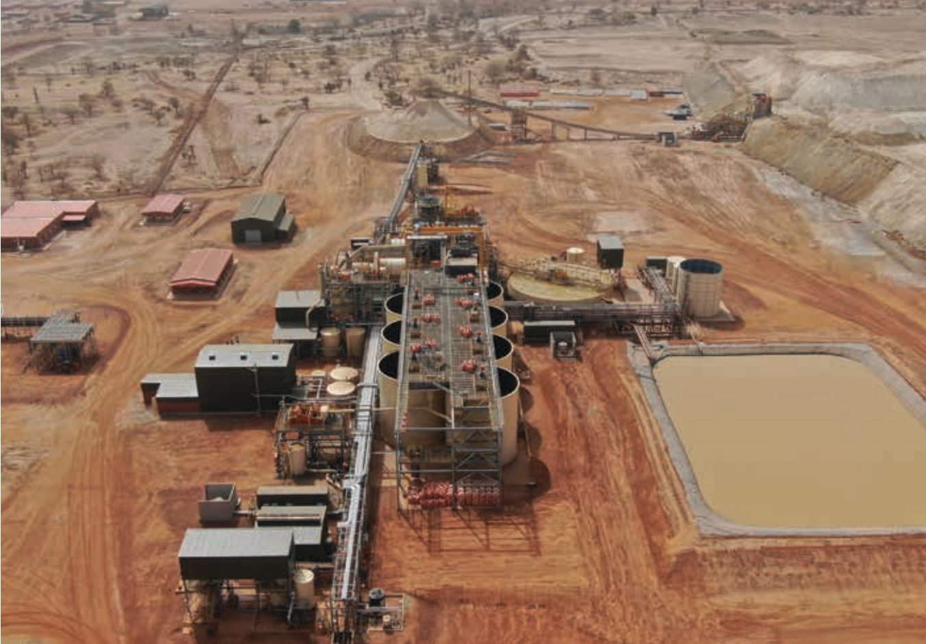
Sanbrado Gold Project, Burkina Faso
