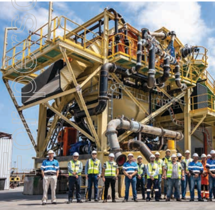
Dry Mining Unit
