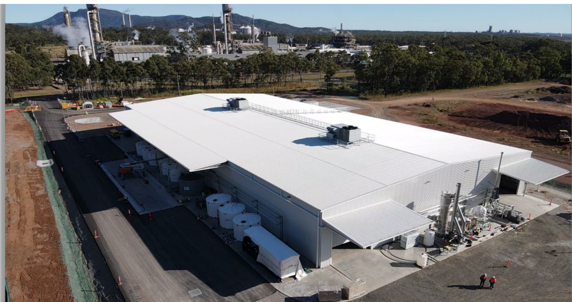
Stage 1 PPF building at lockup stage
