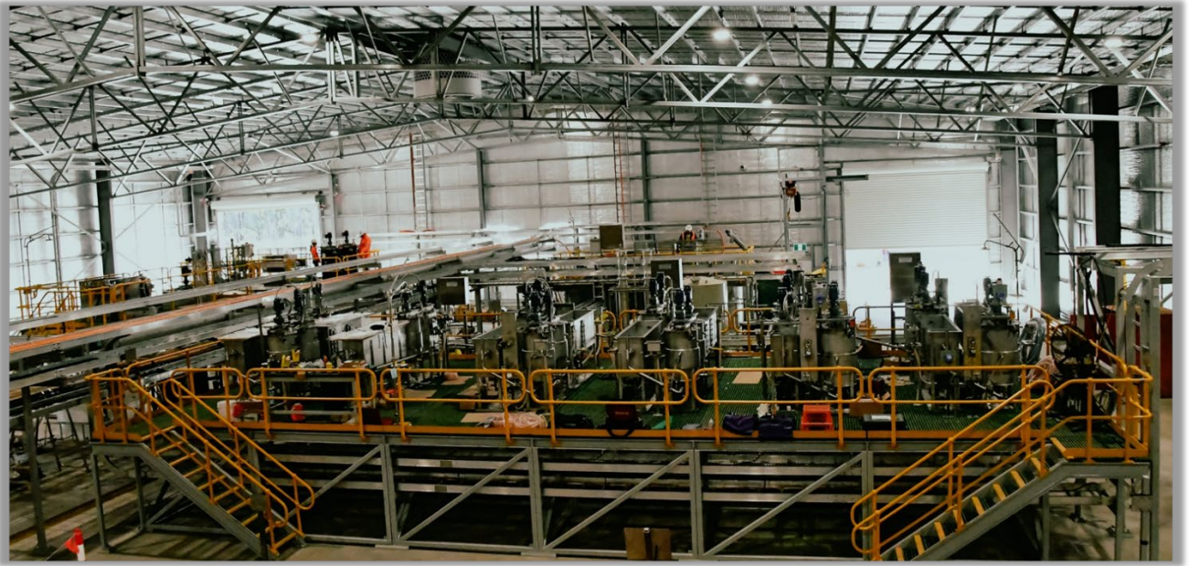
Completed mechanical installation of solvent extraction (SX) circuits
