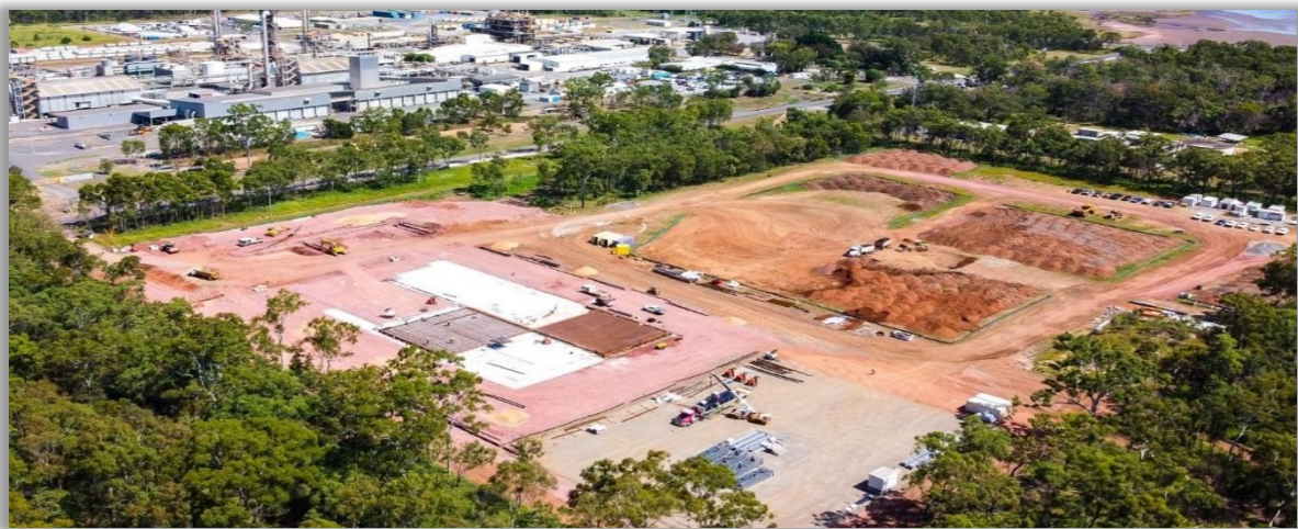
Stage 1 PPF - preliminary earthworks
