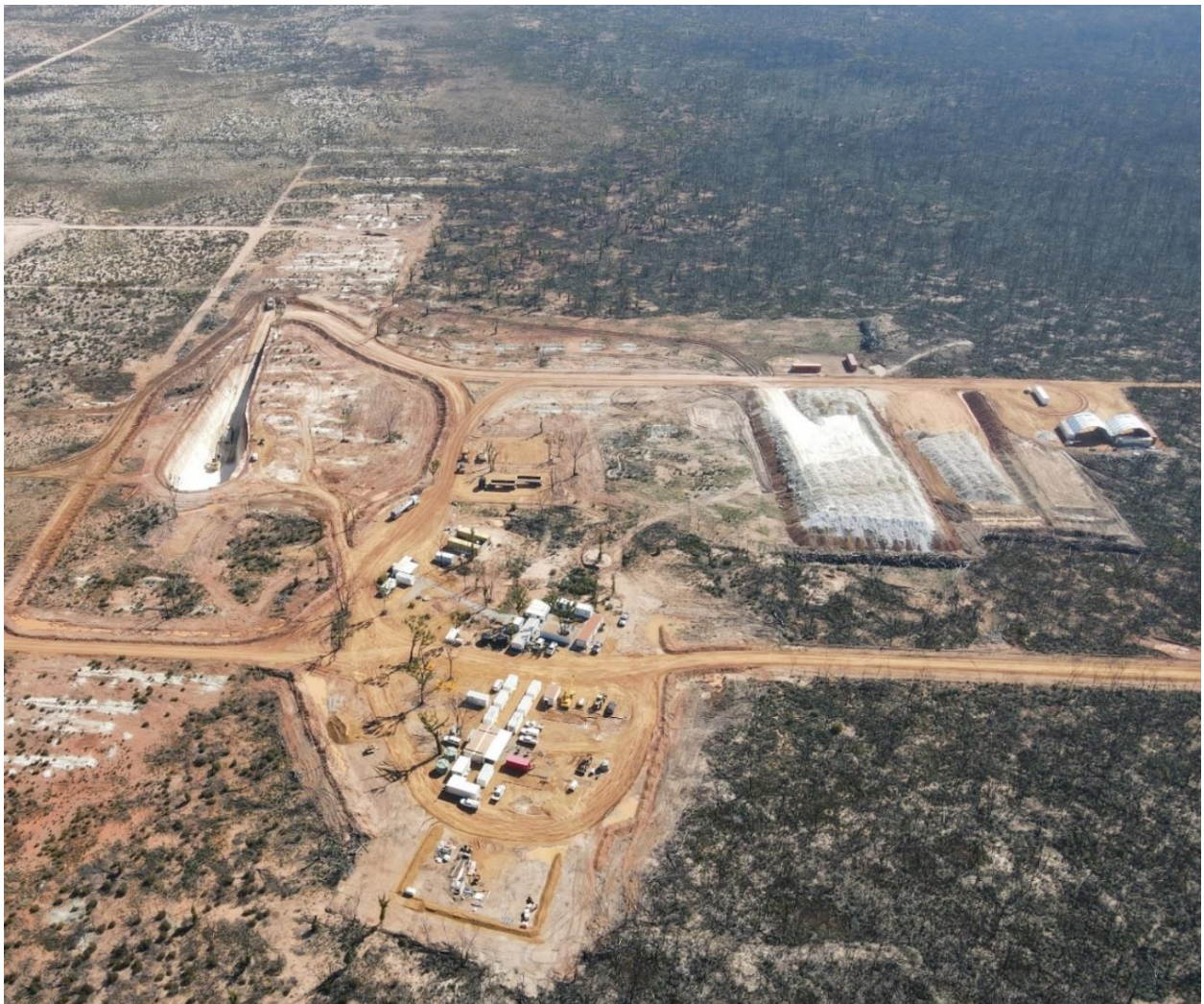
Figure 1: Kat Gap Bulk Sample Pit ready for next stage mining.
