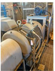
This 600-horsepower electric motor runs at our Bantry 2-29 plant, its role is to increase compression at the facility so produced natural gas can be placed into the sales gas line.
