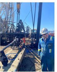
Dustin, one of our wellsite supervisors, is overseeing a workover to convert a previous oil producer to a water disposal well at the 2-29 Bantry Facility. This conversion enables the Company to dispose of additional produced water from our current wells and the recent and future Pisces and Gemini wells. This disposal well is ready to be put in service.
