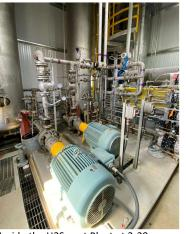
Inside the H2Sweet Plant at 2-29. This facility safely extracts the hydrogen sulphide (H<sub>2</sub>S) from the natural gas and converts it to a solid sulphur cake that can be disposed of safely (or potentially sold with additional processing). This process is one of a kind and reduces operating costs by \$1.30/mcf compared to triazine operations and significantly reduces the comparative environmental impact of triazine disposal.
